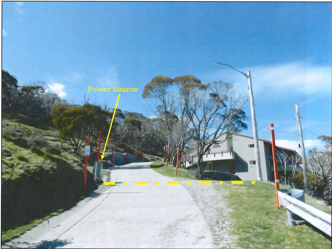
Figure 13. Engineers basic diagram of the proposed underground power route as represented by dashed yellow line
