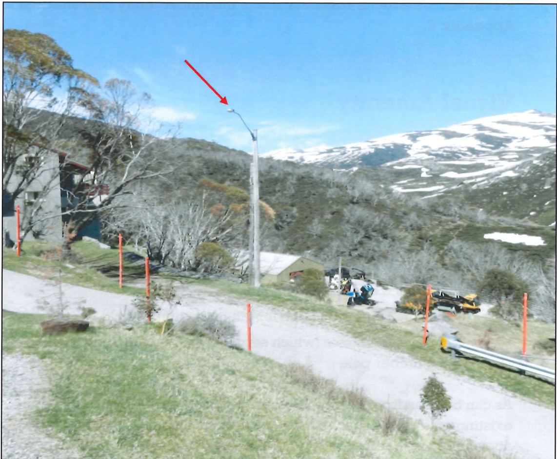
Figure 15. The existing timber light pole and surrounds.
