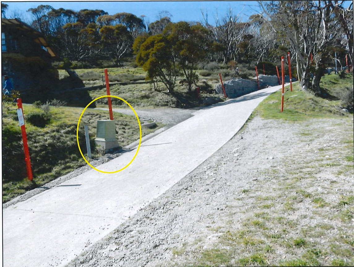
Figure 12. Sealed access within Guthega Village leading to the timber utility pole (timber utility pole located off to the right of the photo). The power box can be seen to the left of the photo (encircled in yellow).
