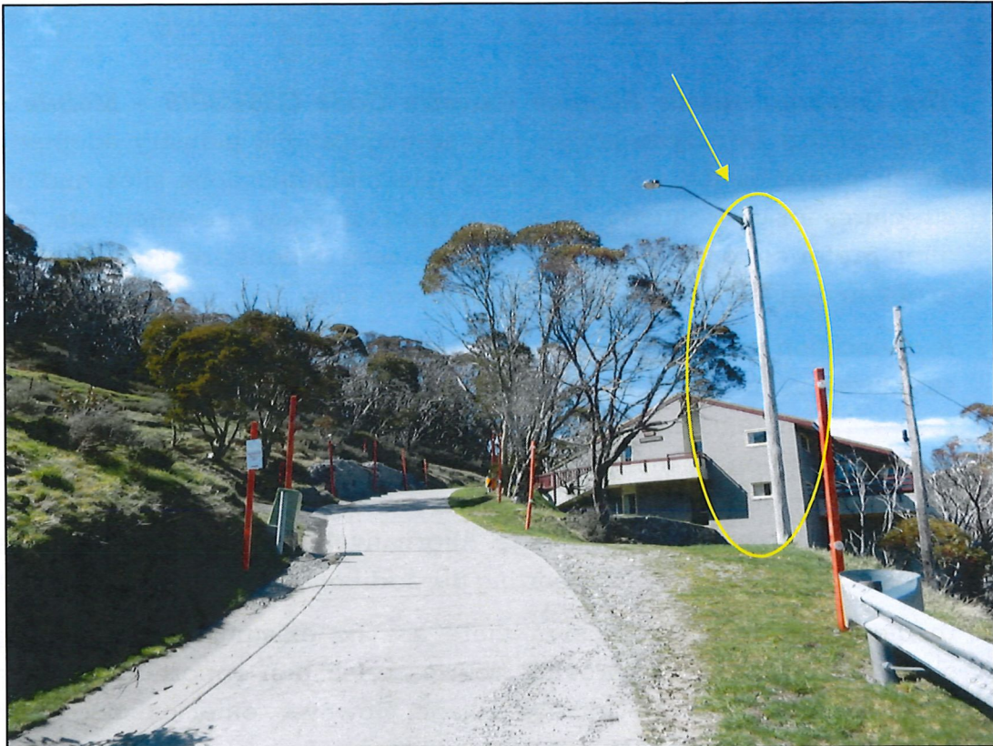
Figure 10. Timber light pole indicated by yellow arrow (view south along Mount Tate Road). The timber pole located to the right was also considered initially, however, was discounted due to rocks in the path of the power route.
